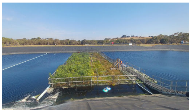
Constructed floating wetlands at Cowes Wastewater Treatment Plant, 2025.
