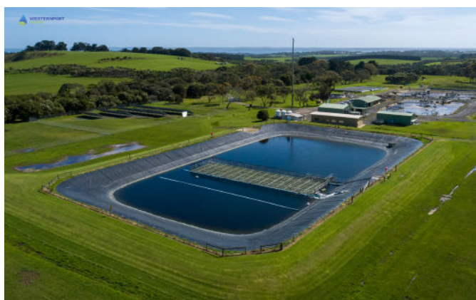
Constructed floating wetlands installed in a treatment lagoon at Cowes Wastewater Treatment Plant.
