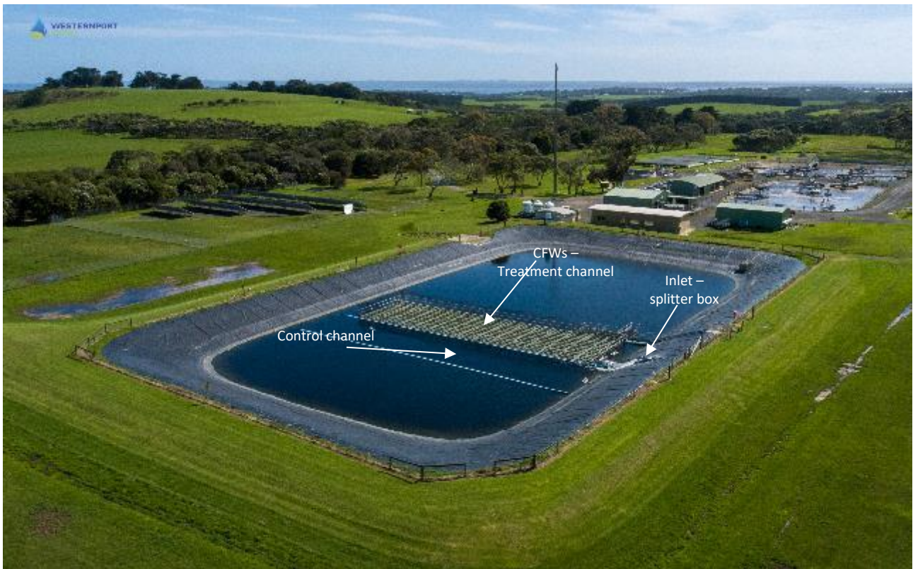
Figure 1. CFWs at the polishing lagoon, Cowes Wastewater Treatment Plant.
