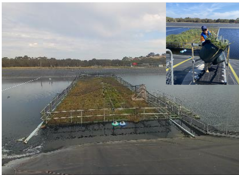
Figure 4. CFWs after plant harvesting. Inset: Harvested plant materials.
