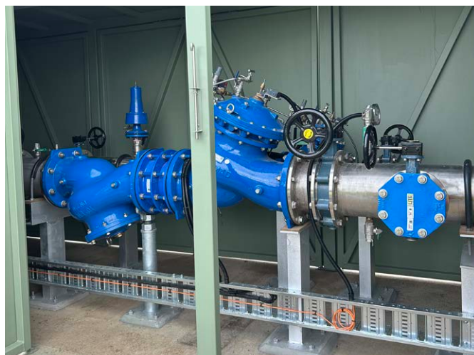
Providing reliable water services with upgrades to the Cowes Pressure Reduction Valve
