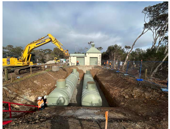
Upgrades to the Rhyll Sewer Pump Station to ensure continuous operation in any weather
