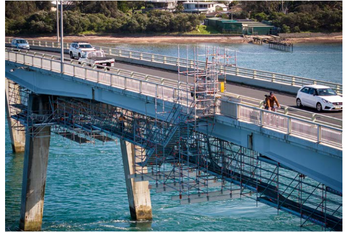
San Remo Bridge upgrades to pipes and fittings
