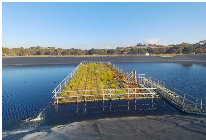
Floating wetlands pilot at the Cowes Wastewater Treatment Plant
