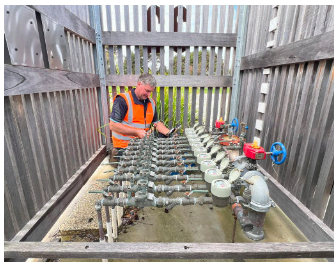
Westernport Water employee demonstrating the backflow testing procedure.
