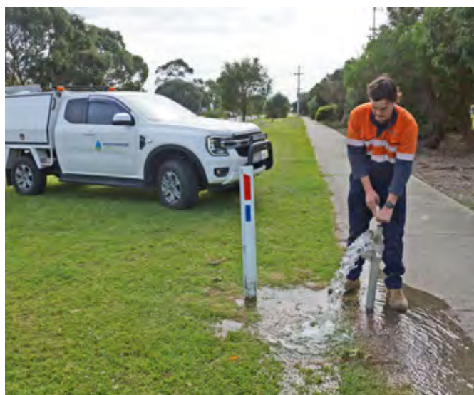
Water mains cleaning is completed annually via air scouring.
