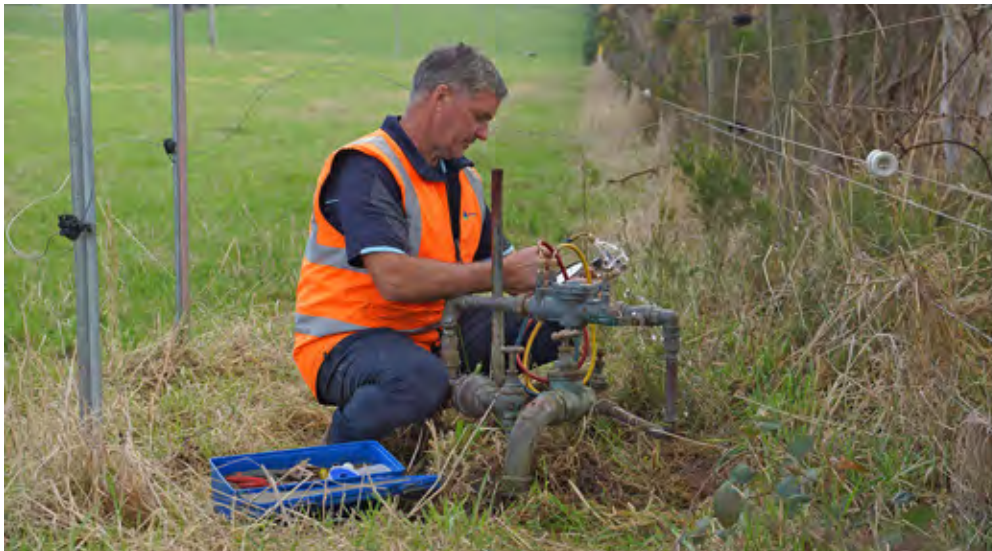
Backflow testing on rural customer water meters.
