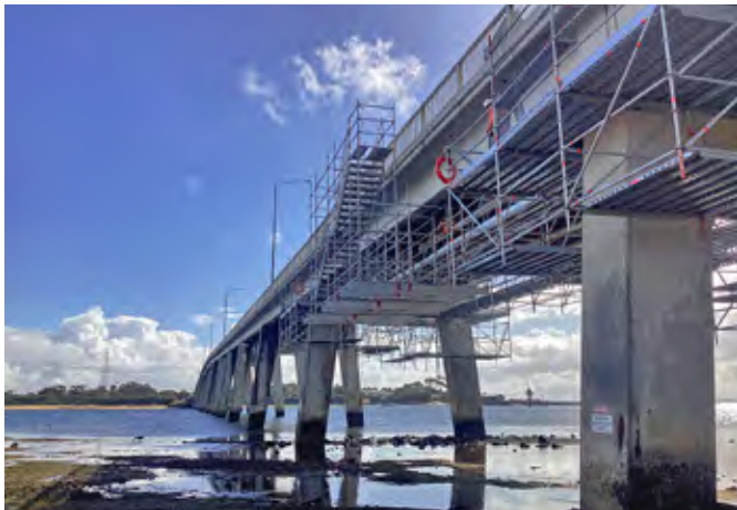
Suspended scaffolding allows workers safe access to the underbridge pipelines while minimising impacts to traffic and pedestrians.
