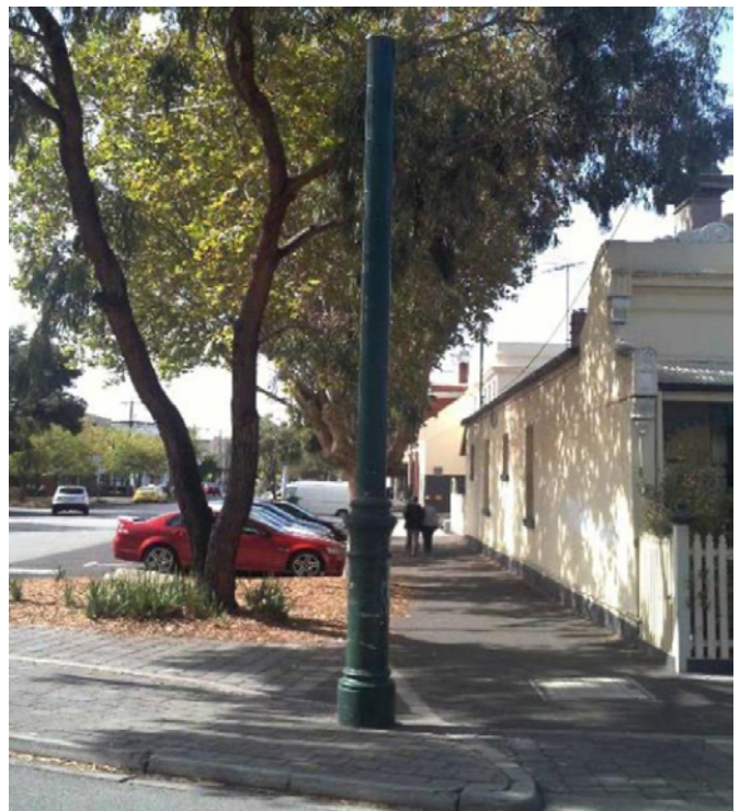
Figure 13: Sewer vent shaft
