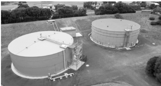
The Phillip Island Water Security Project saw the construction of a new 2.3ML back-up water tank to improve water reliability to Phillip Island customers
