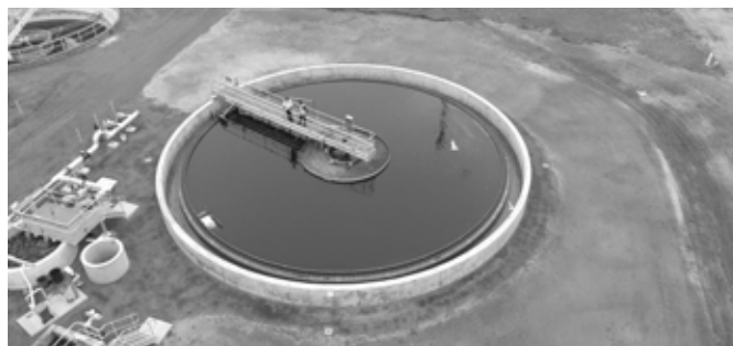
The Cowes Wastewater Treatment Plant was upgraded with a new clarifier to improve performance and meet future growth
