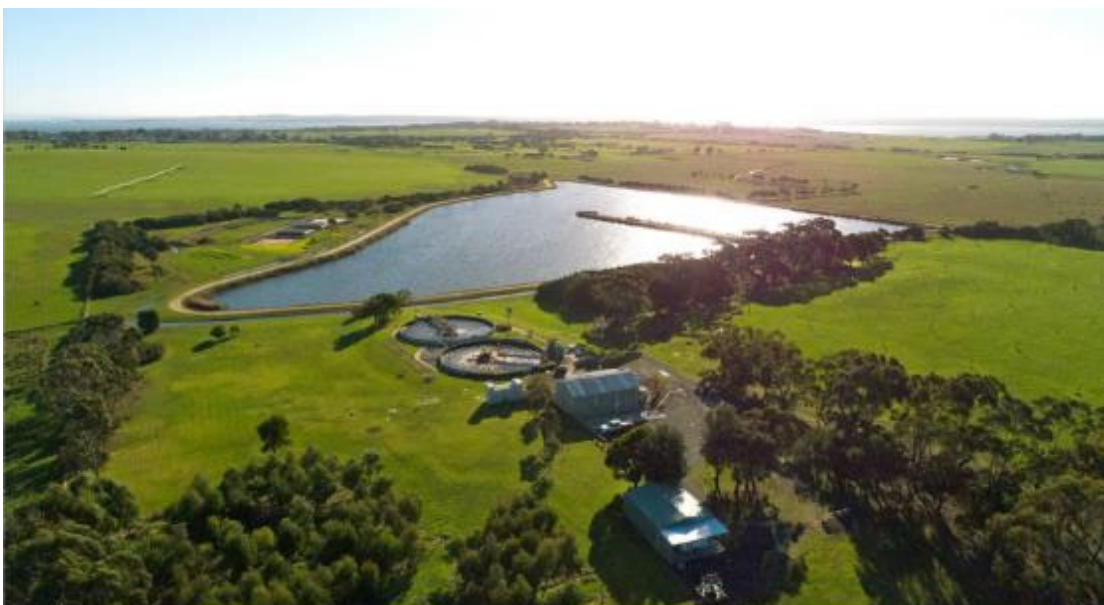
Figure 1 King Road Waste Water Treatment Plant
