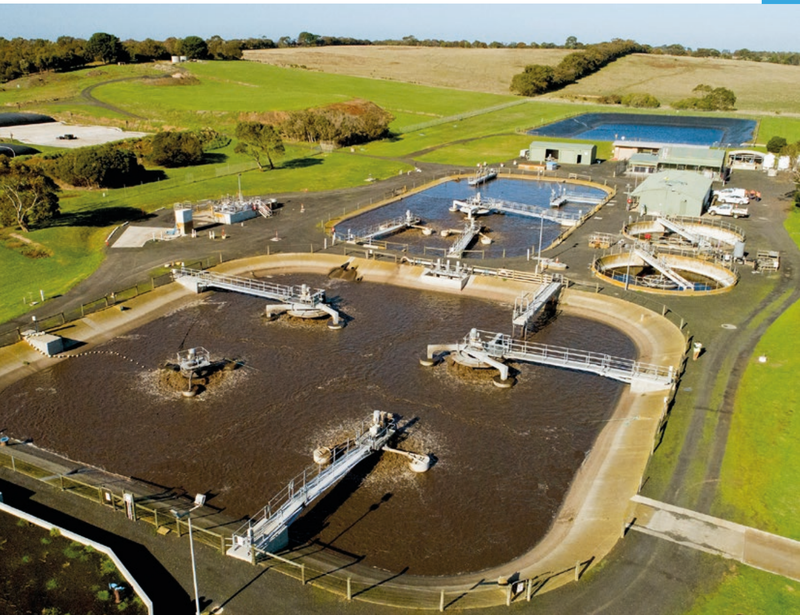
Photo description: Cowes Waste Water Treatment Plant.
