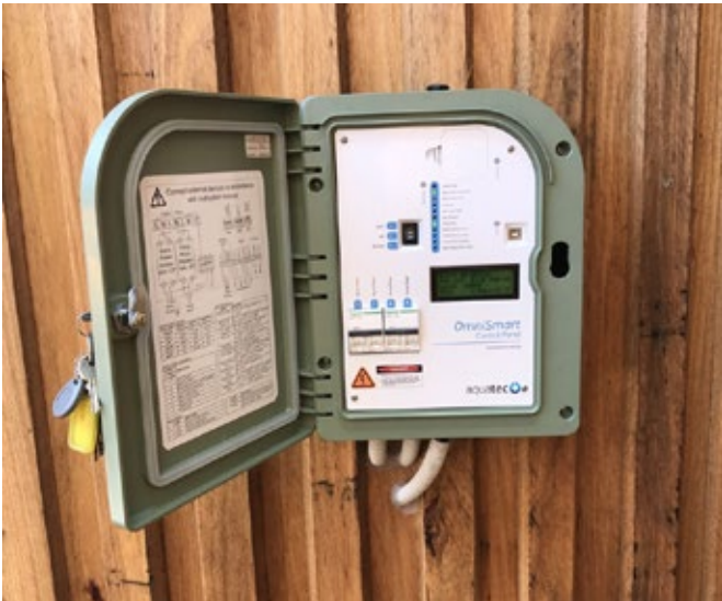
Figure 14 – Pump Control Box
