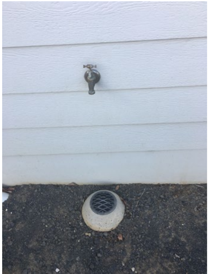
Figure 31 – Overflow Relief Gullies
