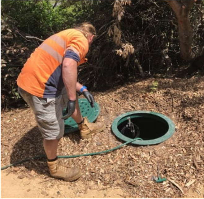
Figure 13A – Tank Unit after Installation
