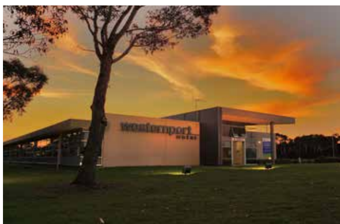
Above: Westernport Water Head Office.
