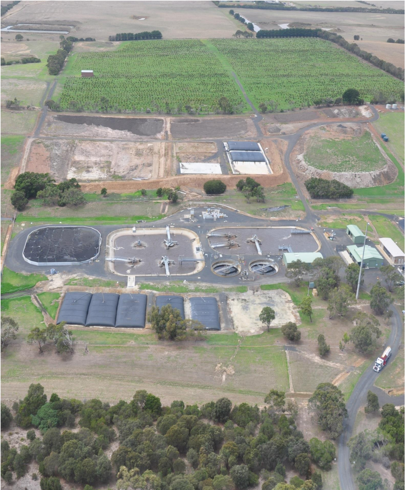
Cowes Waste Water Treatment Plant – 2016
