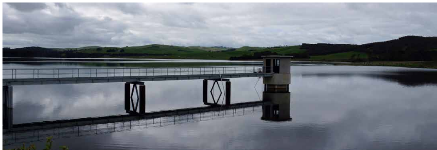
Candowie Reservoir Water Tower
